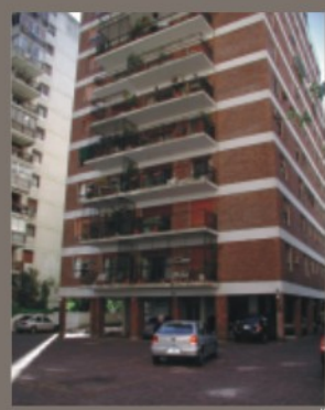
The Reinforced Concrete Tomography is used to study balconies in apartment buildings.
